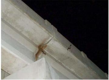
Photo 7: Staining along longitudinal joint. Note Photo 8: Staining on underside of expansion joint from bat use. guano deposits on the ground.
