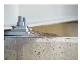
Photo 5: Guano deposit on pier, obscuring structural features.
